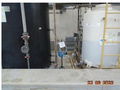
ABPR3_Chemical dosing (Cooling Tower 30)
